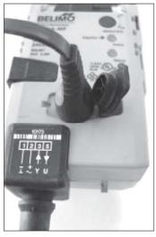
AR, GR, LR, NR, AK, GK Series Use the interface on the top of the actuator. (Leave all of the wires of the actuator installed.)
